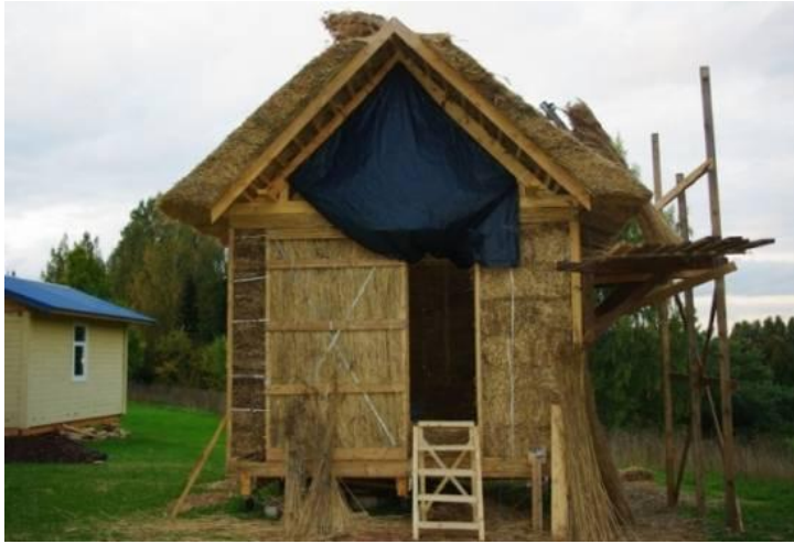
Figure 3.2. a Wall VS-1 (vertically laid reed wall)
