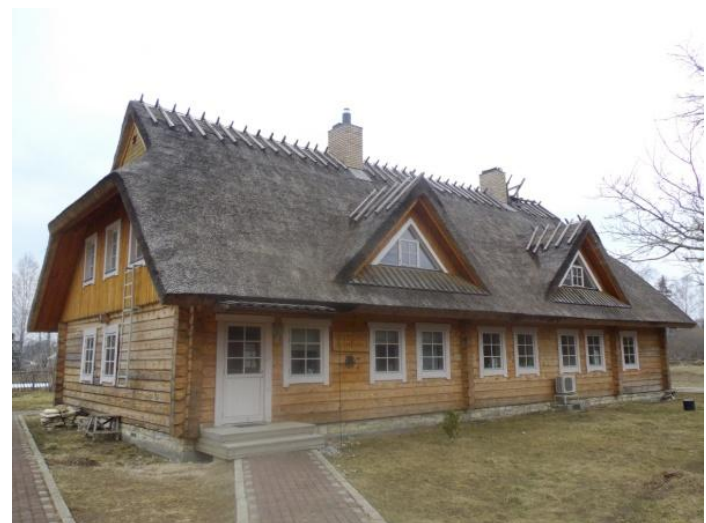
Some pictures of investigated dwelling houses (Photos: S. Sõber)
