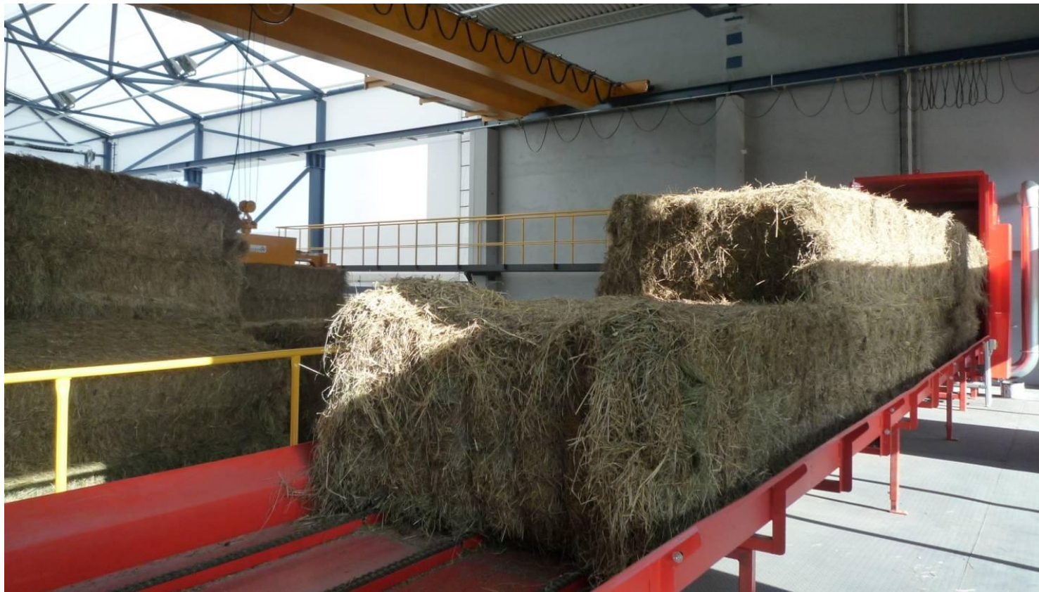
Figure 4.8. Hay (left) and reed (right) on a conveyer belt at Lihula Boiler House (Photo: Ü. Kask)
