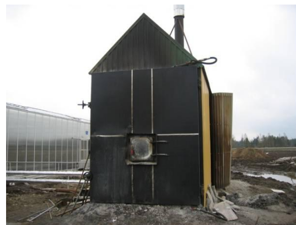
Figure 4.6. Boiler for burning round and square grass and straw bales (Photo: Ü. Kask)
