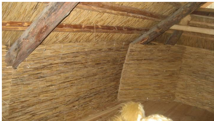
Figure 3.43. Properly insulated attic (Photo: S. Söber)
