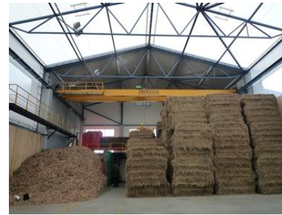
Figure 5.13. Storing of large square bales in Lihula (Estonia) boiler house storage (Photo: Ü. Kask)
