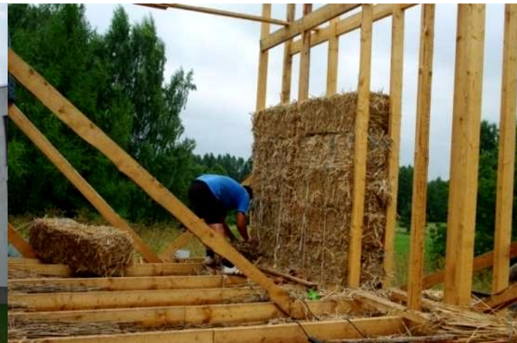
Figure 3.2. d Wall VS-4 (reed block wall)
