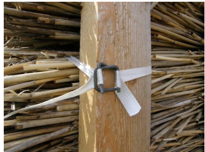
Figure 3.23. Fixing of loose reed with plastic straps in wall VS-2 (Photo: J. Miljan)
