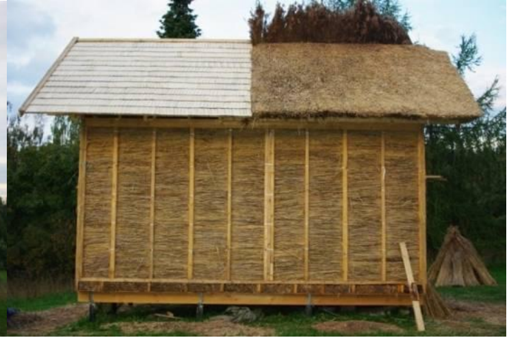
Figure 3.2. b Wall VS-2 (horizontally laid reed wall)
