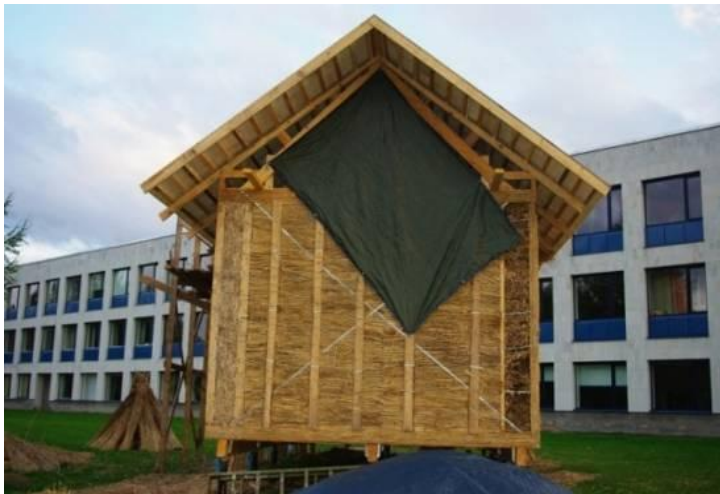
Figure 3.2. c Wall VS-3 (reed panel wall)
