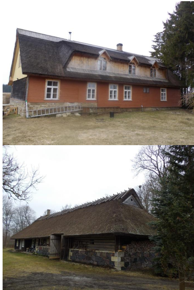
Figure 3.38. Farms studied. Upper: thatched roof with ridge covered with aspen boards and lower: the hip roof with venny holes and traditionally reinforced ridge (Photos: S. Söber)
