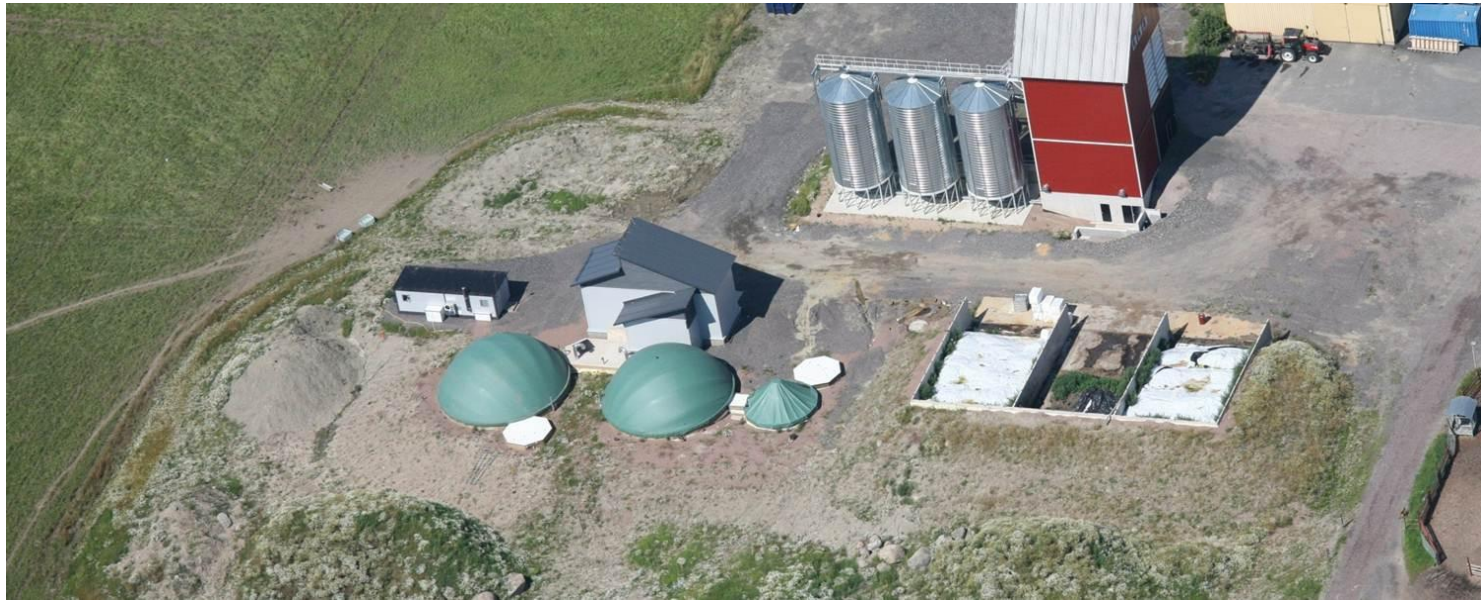
Figure 6.6. The biogas plant at Livia College
