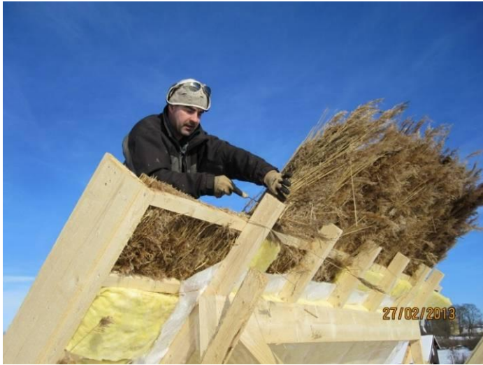
Figure 3.34. Veli-Matti Saaren-Kierola cutting the reed stalks going over the ridge.
